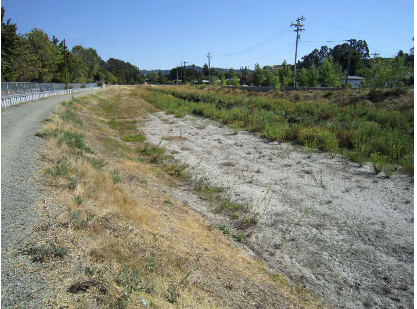
Figure 8. Pinole Creek #3 Assessment Area, looking upstream. Note the barren (foreground) and mowed (background) condition of the floodplain surface.
