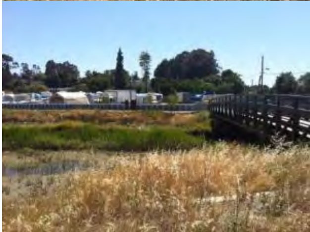
Photopoint 2 (2011) upstream, downstream, across stream
