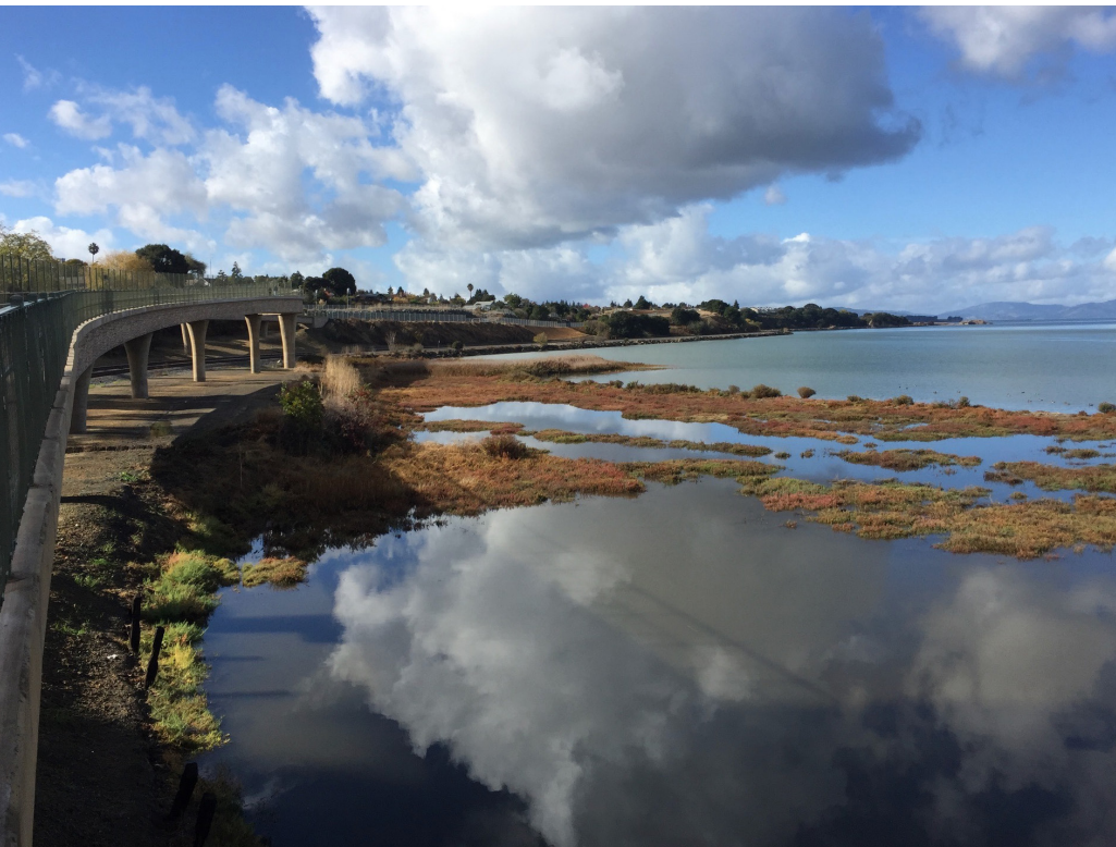
The Bay Trail bridge over the rail road tracks along Bay Front Park greatly enhances the Pinole Creek trail and experience.
