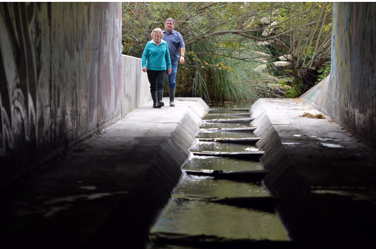
FOPCW Co-founder Carol Arnold and Board member Bert Mulchaey walk inside the newly renovated fish passage on Pinole Creek. The old box culvert, which prevented fish from spawning upstream, was removed with the help of the Friends of Pinole Creek.
