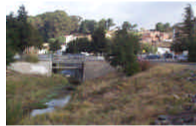
Flood control channel entering a concrete box culvert
