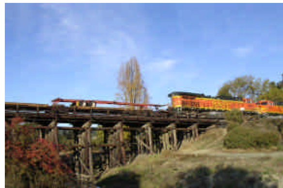
The Sante Fe Railroad crosses Pinole Creek on a historical trellis bridge
