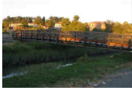
New footbridge crossing near the bay trail
