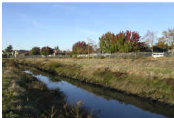
The lower portion of Pinole Creek with private property in the background
